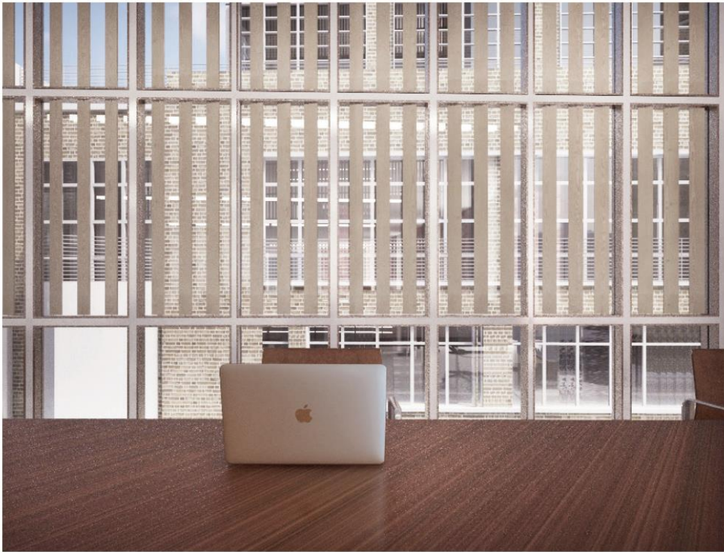
Position 2 Level 5 Standing - Upper panels Type A louvres; Lower two panels Type B (left) and Type C (right)
