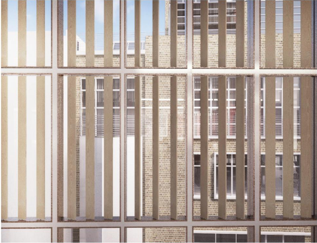
Position 3 level 4 Sitting – Upper 2 panels Type B louvres, Lower panel Type C louvres
